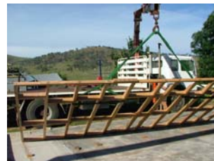
Our crane truck in action standing up a house frame.
